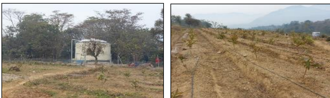
Figure 15: Main water tank & Drip Irrigation System
