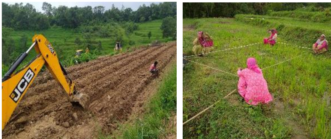
Figure 12: Site Clearance for plantation
