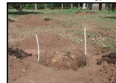
Preparation of Pit
