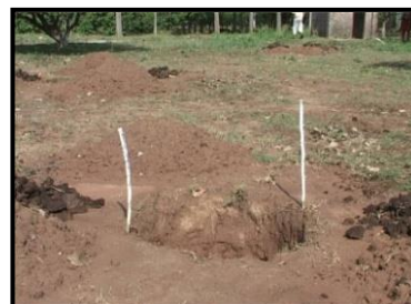
Preparation of Pit
