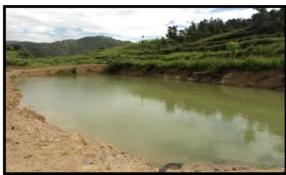
Water Harvesting Pond
